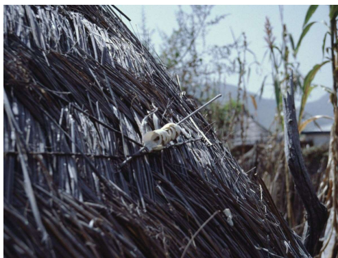
Photo 29: Egg shells lined up on the roof.
