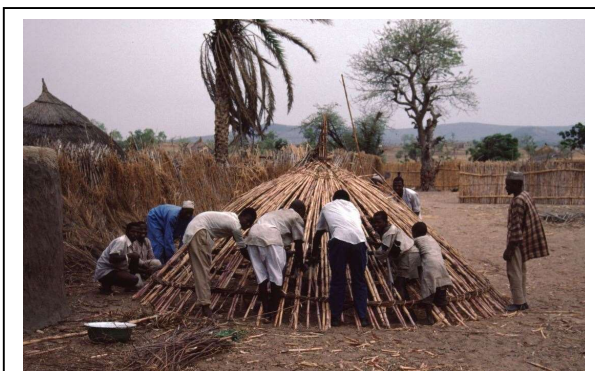
Photo 25: Building a house roof.
