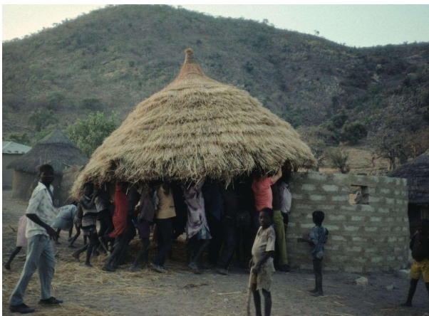
Photo 10: Attaching the roof to a new house
