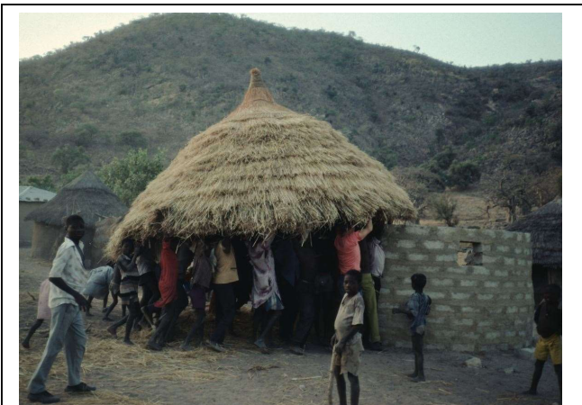
Photo 10: Attaching the roof to a new house
